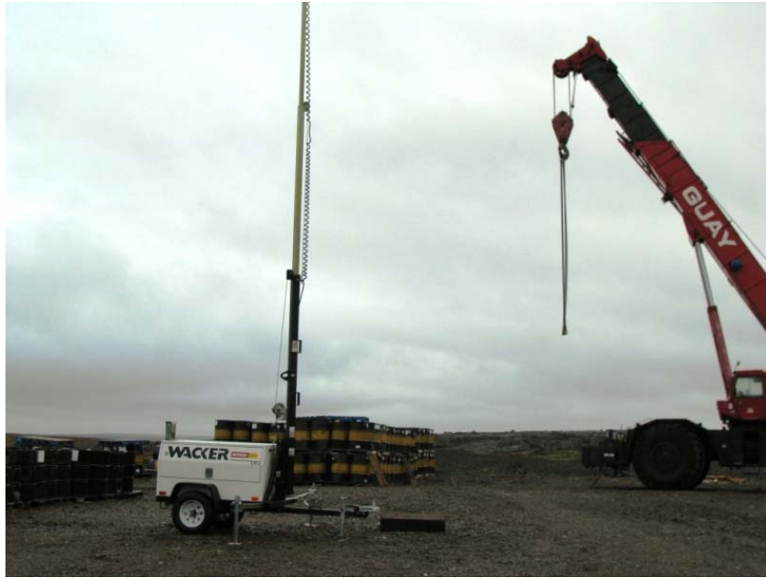
Photo 5: Fuel storage at Nova Camp.
