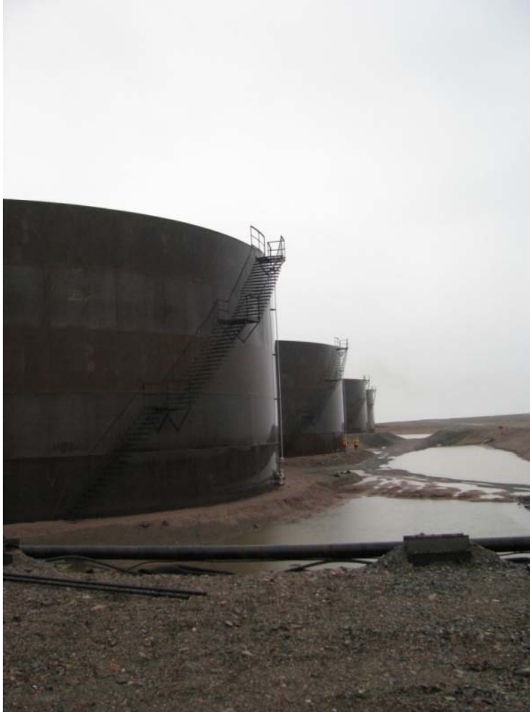
Photo 9: Baker Lake fuel tank farm.
