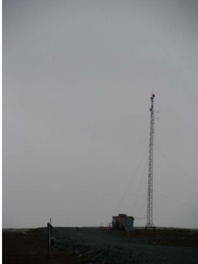
Photo 3: Communications tower at kilometre 37.
