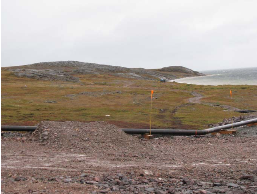
Photo 1: ATV crossing at Baker Lake fuel storage and barge landing facility.
