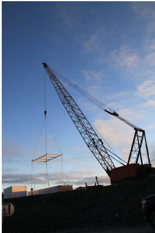
Photo 12: Construction of new kitchen facilities
