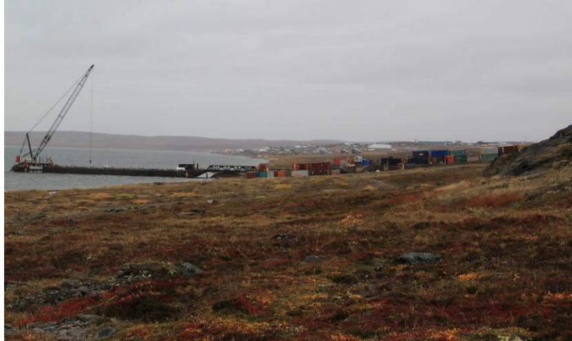
Photo 30: Baker Lake barge laydown facility (photo taken September 17, 2011)
