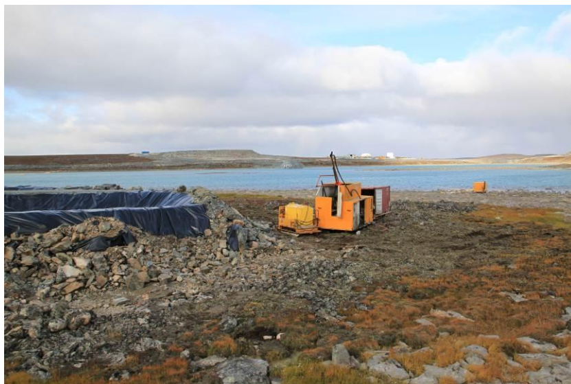
Photo 13: Drilling of groundwater well at Bay Goose area
